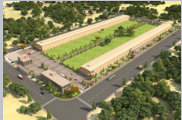
Jaipur Plant, India
